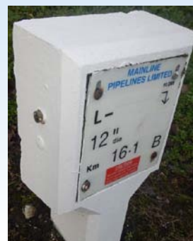
Beware of posts with brass studs (such as the post above) which have cables connecting to the pipeline below.
