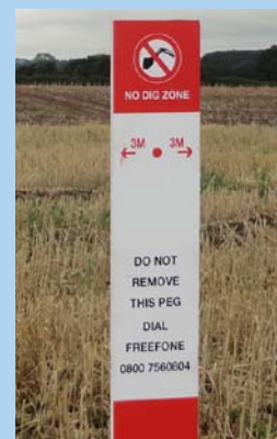
When the pipeline route has been located it will be marked with location pegs.
