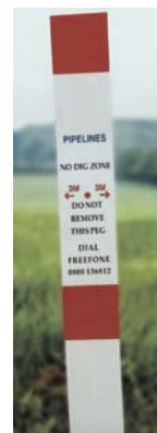
When the pipeline route has been located it will be marked with location pegs.
