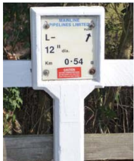
Mainline marker post
